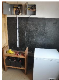
Ongoing installation of command center and refrigerator
